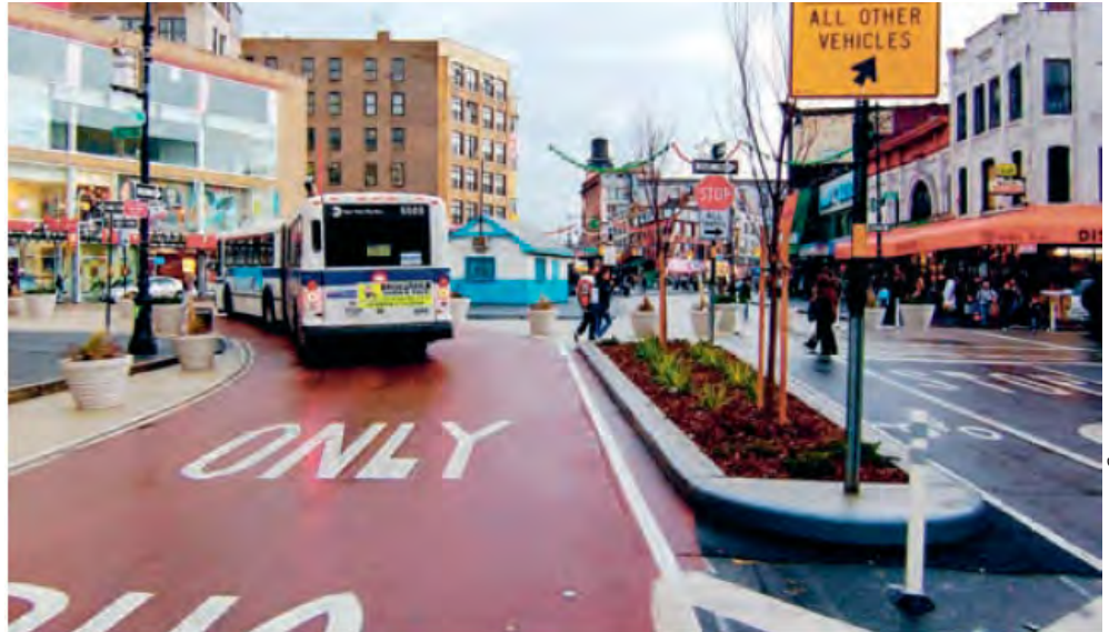
Bus lane separated from bicycle and motor vehicle lanes by a median that also serves as a pedestrian refuge in New York City
