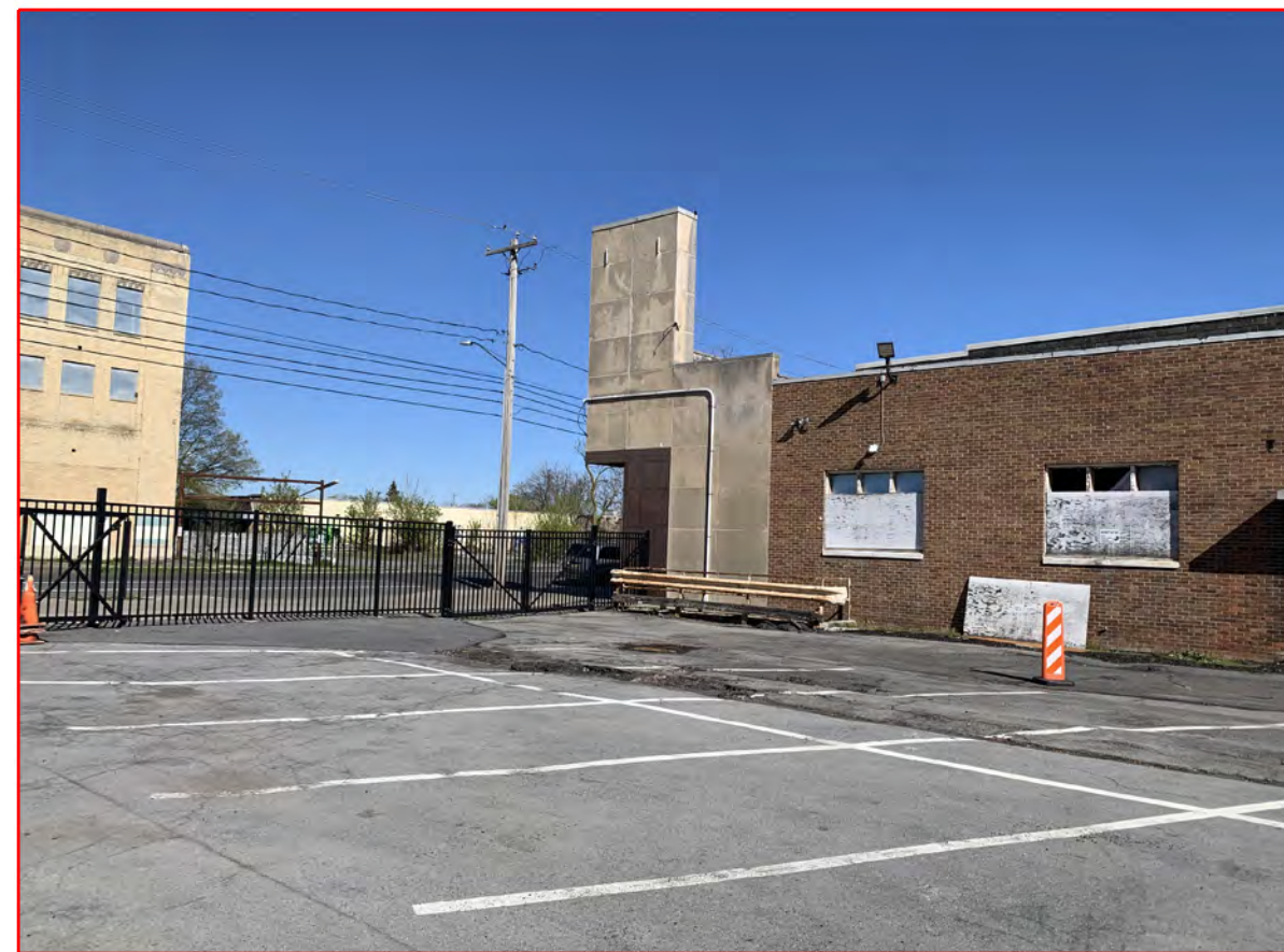
PHOTO: 1 - 1227 SOUTH SALINA STREET (VIEW: NORTHWEST)
