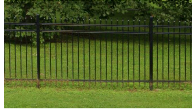
SITE FENCING / GATES
