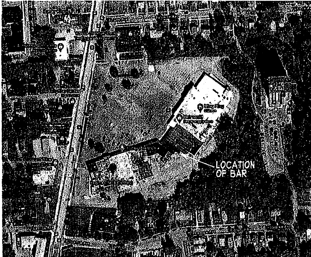
Figure No. 2: Aerial photo of Valley Plaza from Zoning Application (see Exh. 1, p. 6)
