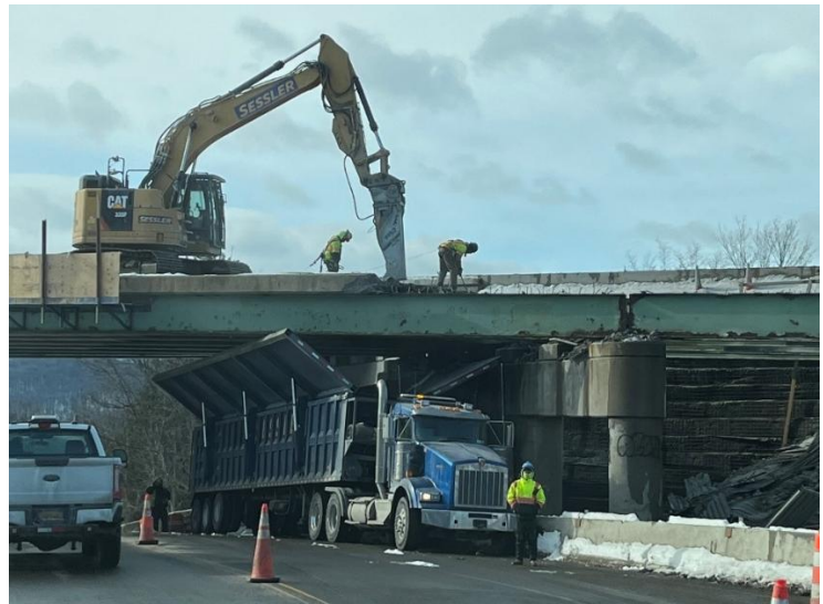
Pictures of Route 81 project construction in progress
