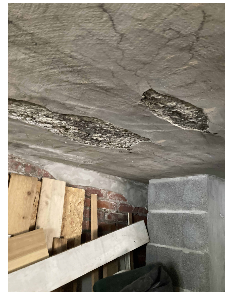
PHOTOS OF EX. CONC. SLAB FAILING*
