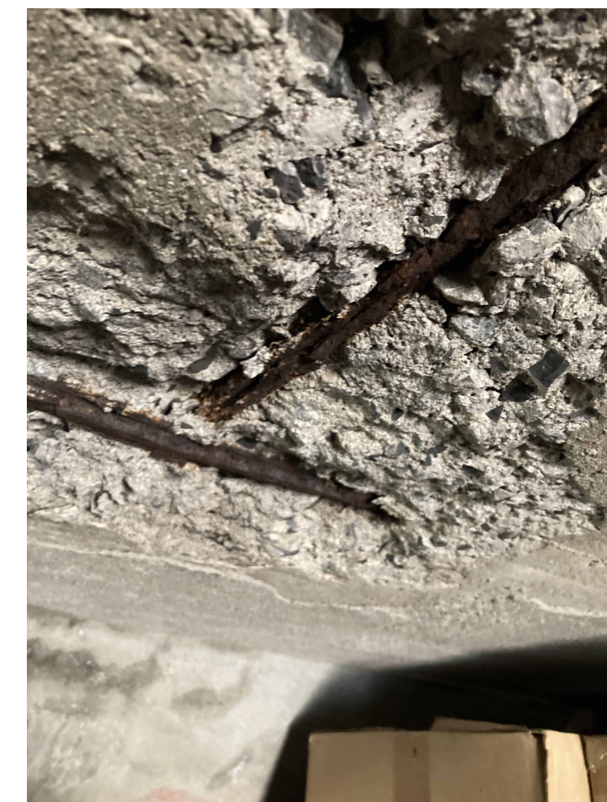
PHOTOS OF EX. CONC. SLAB FAILING*
