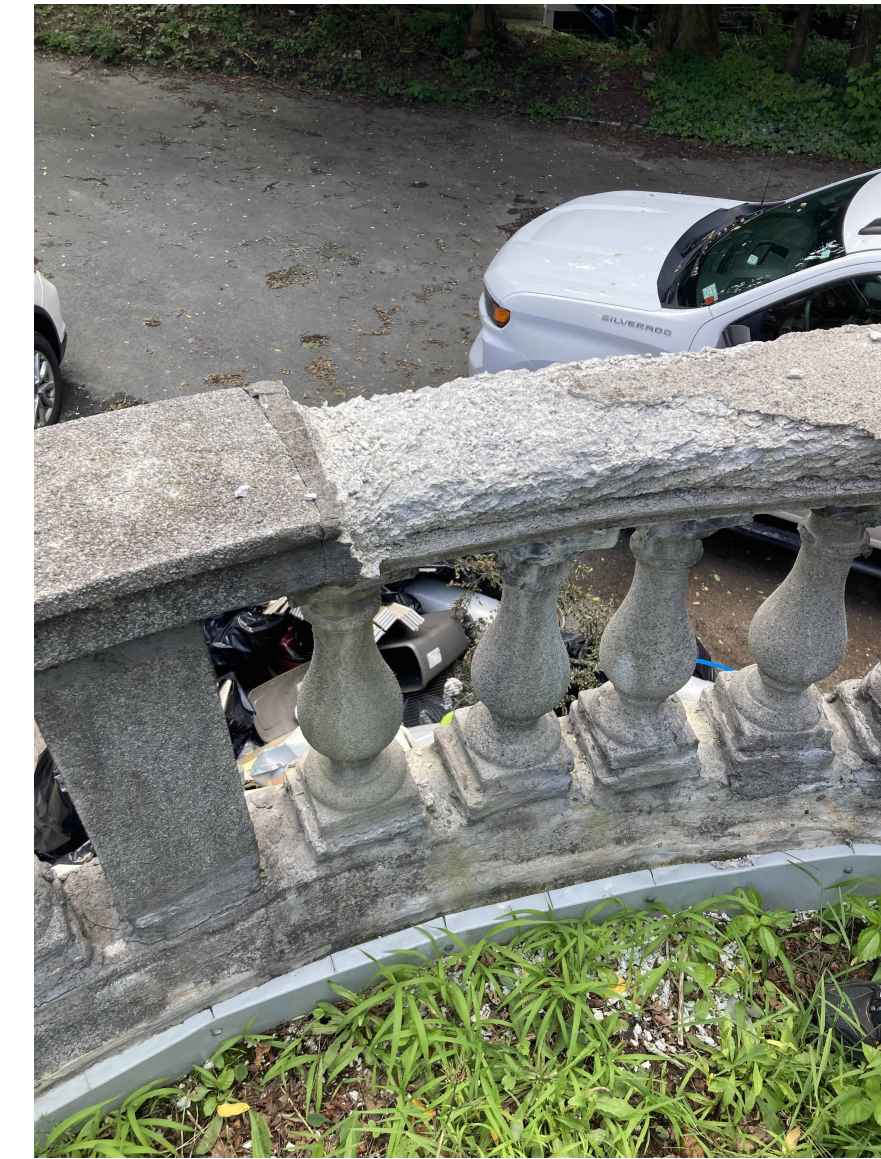
PHOTOS OF EX. BALUSTERS DETERIORATING*
