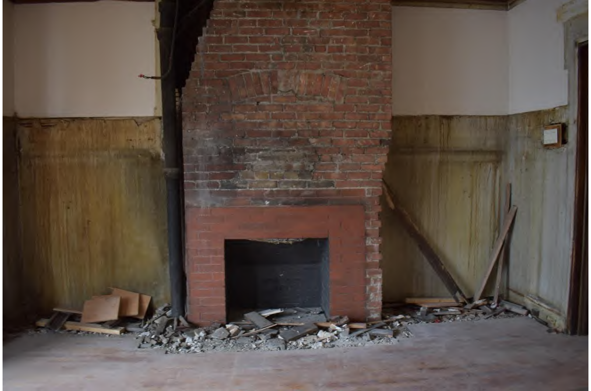
24. View of the fireplace in the dining room. All wood details and mantel pieces have been removed.
