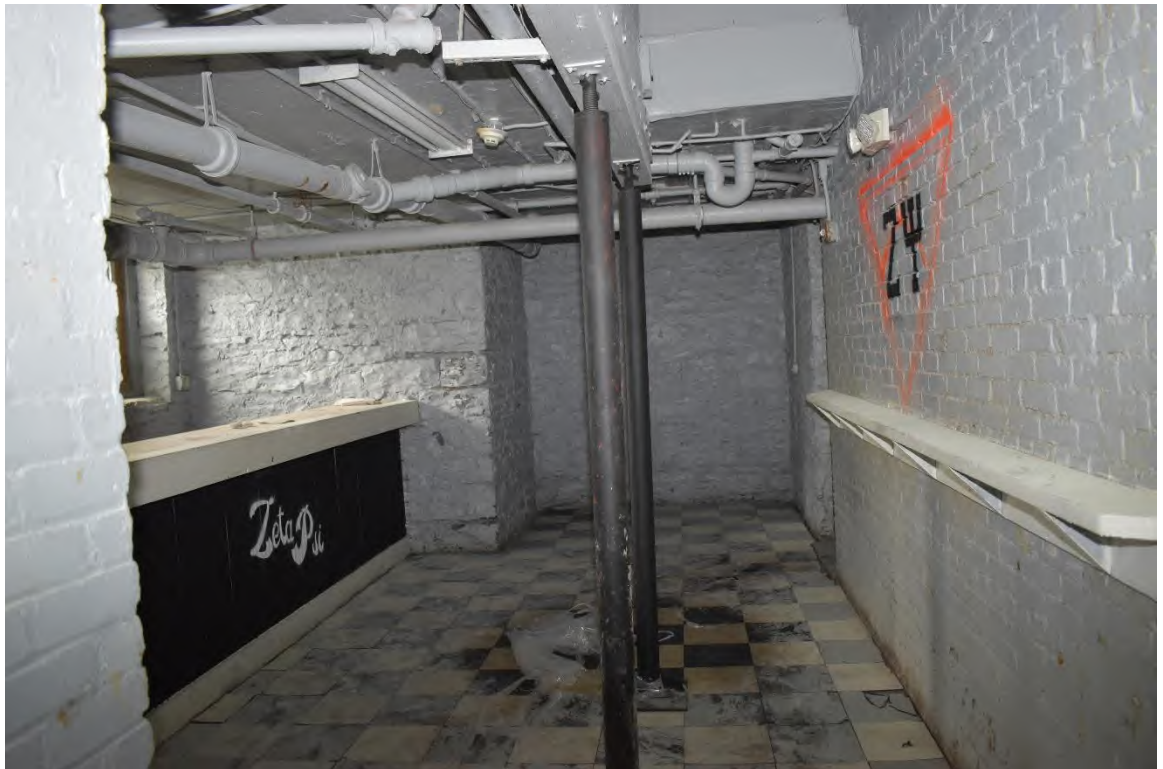
35. The bar is located in the northern portion of the basement.
