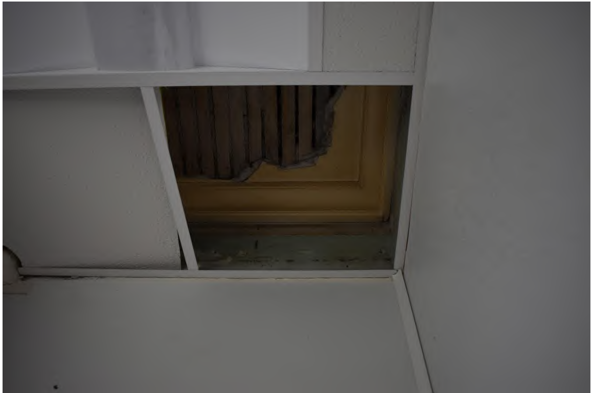
45. The bathrooms include drop ceilings that hide original ceiling details.
