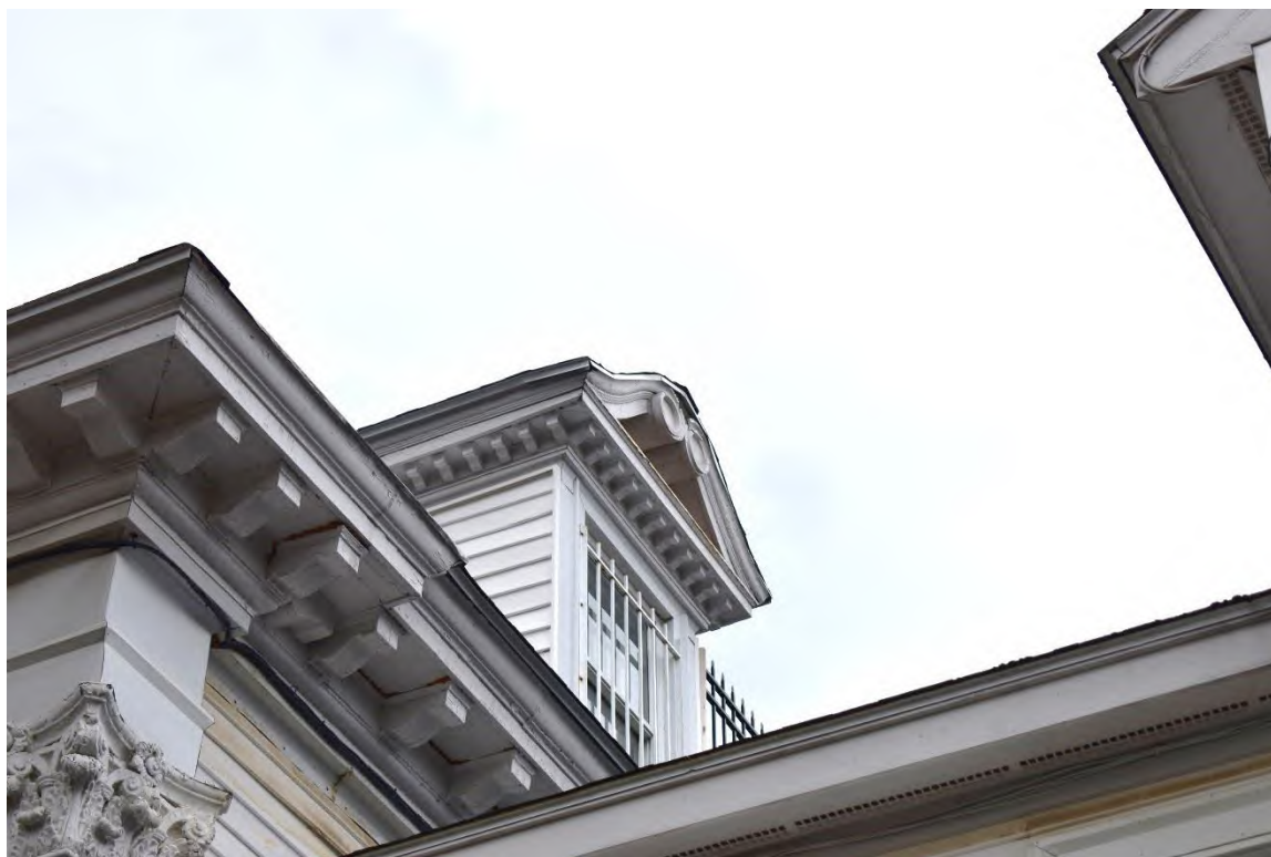
13. Detail view of the dormers on the eastern elevation.
