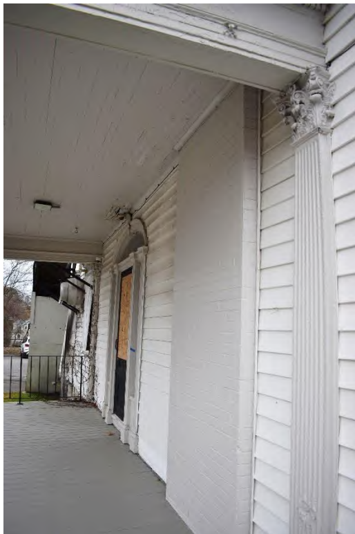
15. Detail view of the veranda and entrance on the northern elevation.
