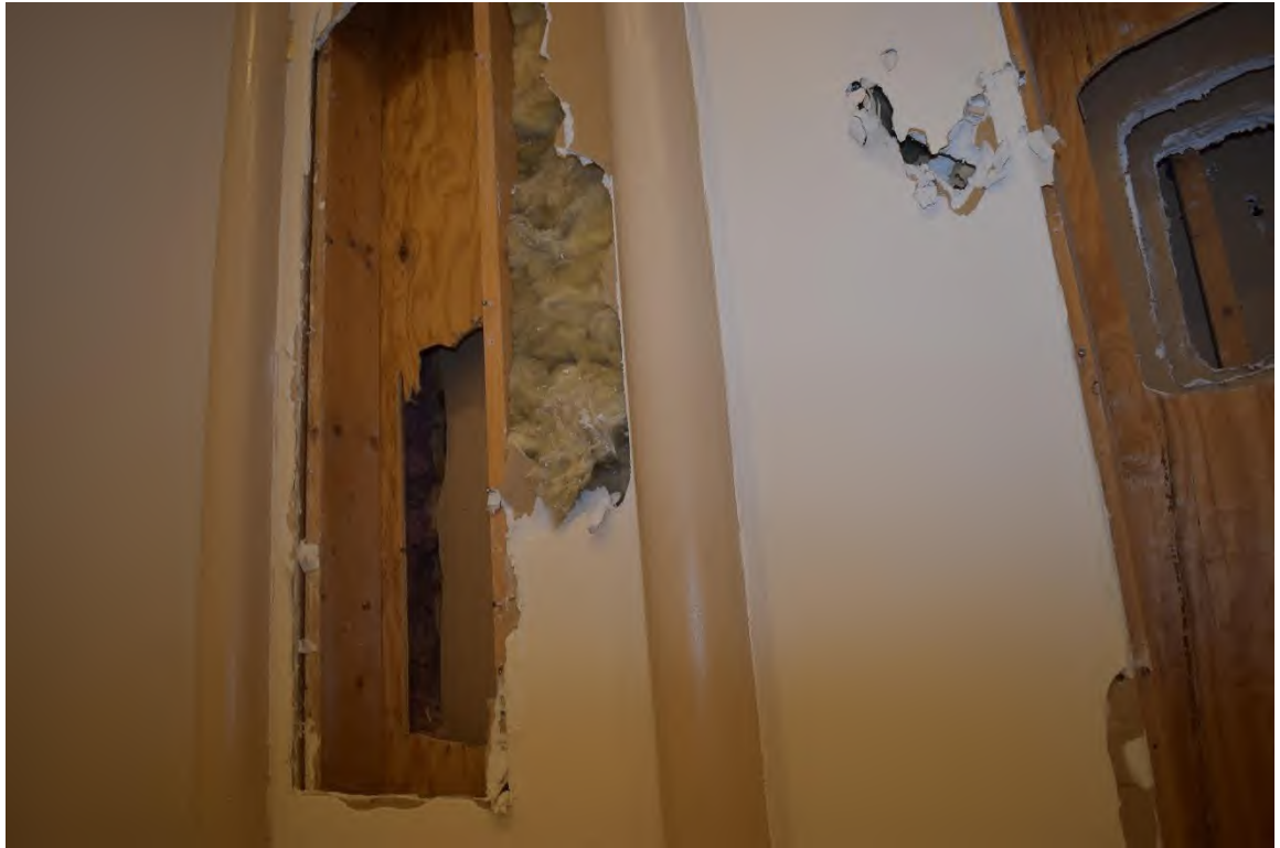
29. Openings in the wall show numbers renovations with modern building materials.
