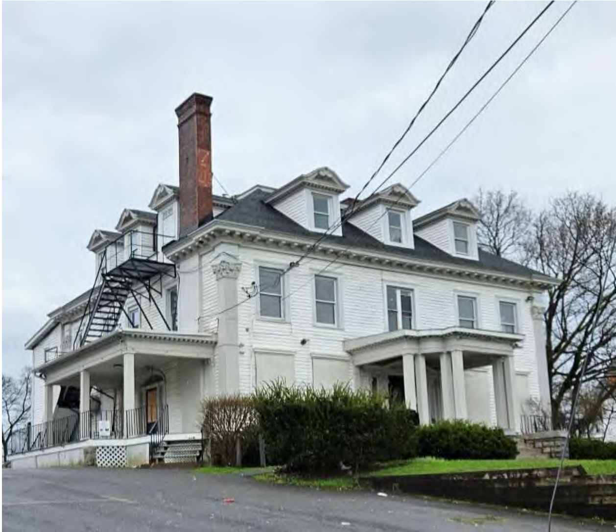
Photo 1: View to the southeast of the façade of 727 Comstock Avenue. The entrances are marked by decorative porches.
