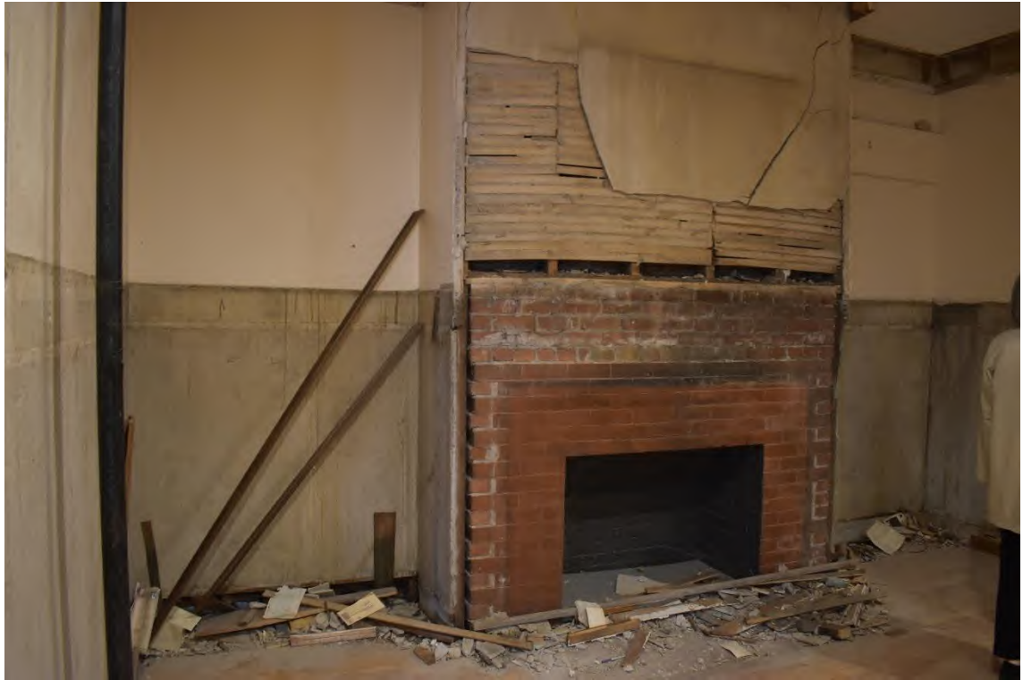
22. View of the fireplace in the library. All wood paneling and mantel details have been removed.
