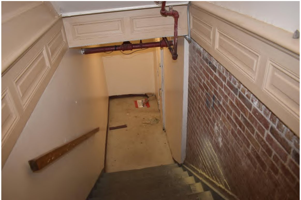
37. View down the main stairwell to the basement.
