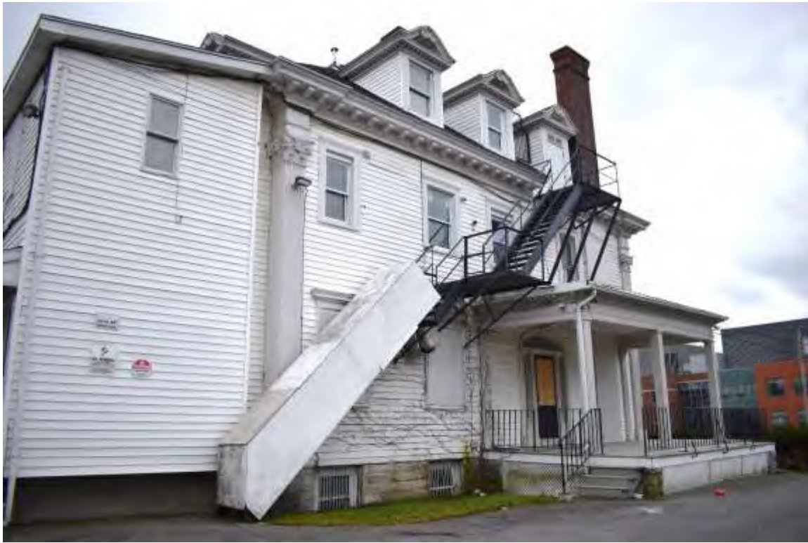
Photo 2: The northern elevation features an emergency access ladder over the northern portion. View to the southwest.
