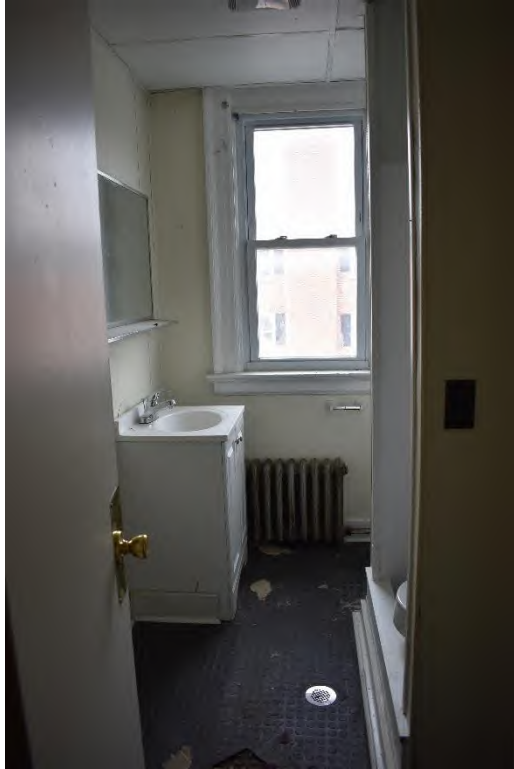
44. View of the bathroom on the second floor.
