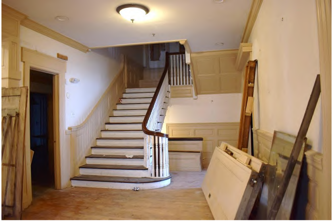
19. View of the foyer and main staircase.
