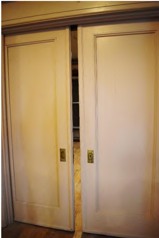
23. Library entrance features pocket panel doors.
