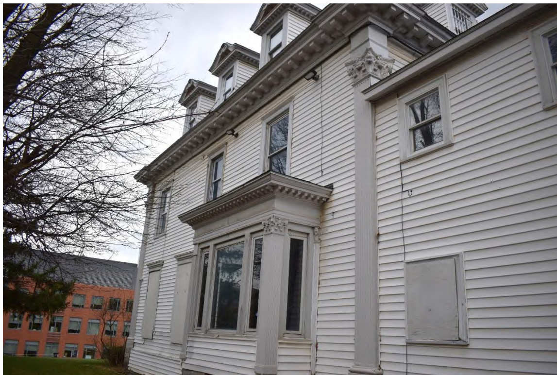
12. View to the northwest of the southern elevation.
