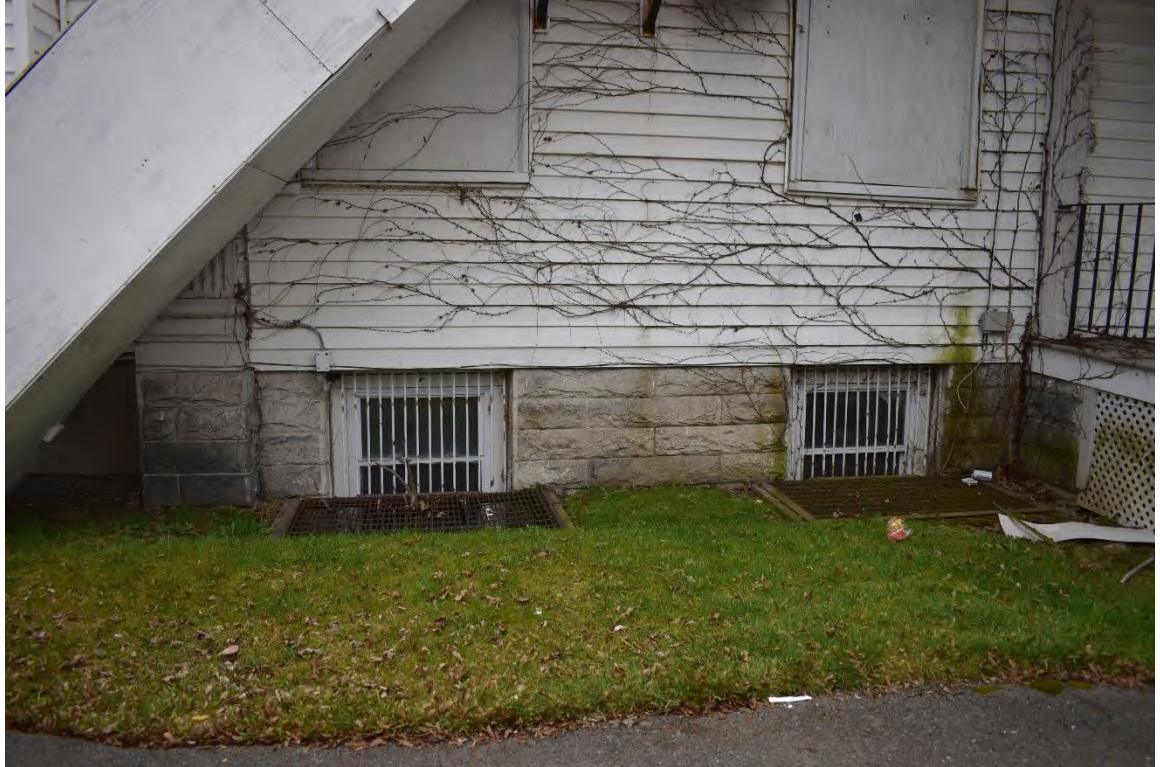
16. Detail of window wells for basement bar on northern elevation.
