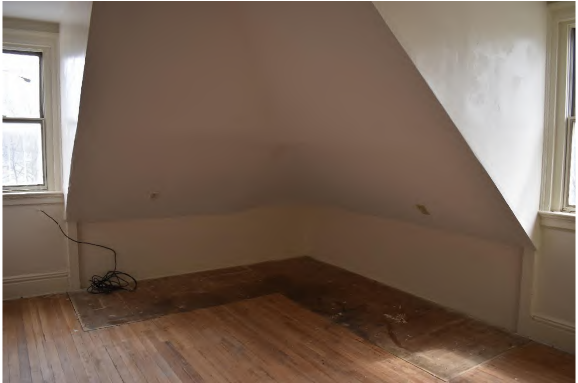
47. View of a 3 rd floor bedroom (Room 304)
