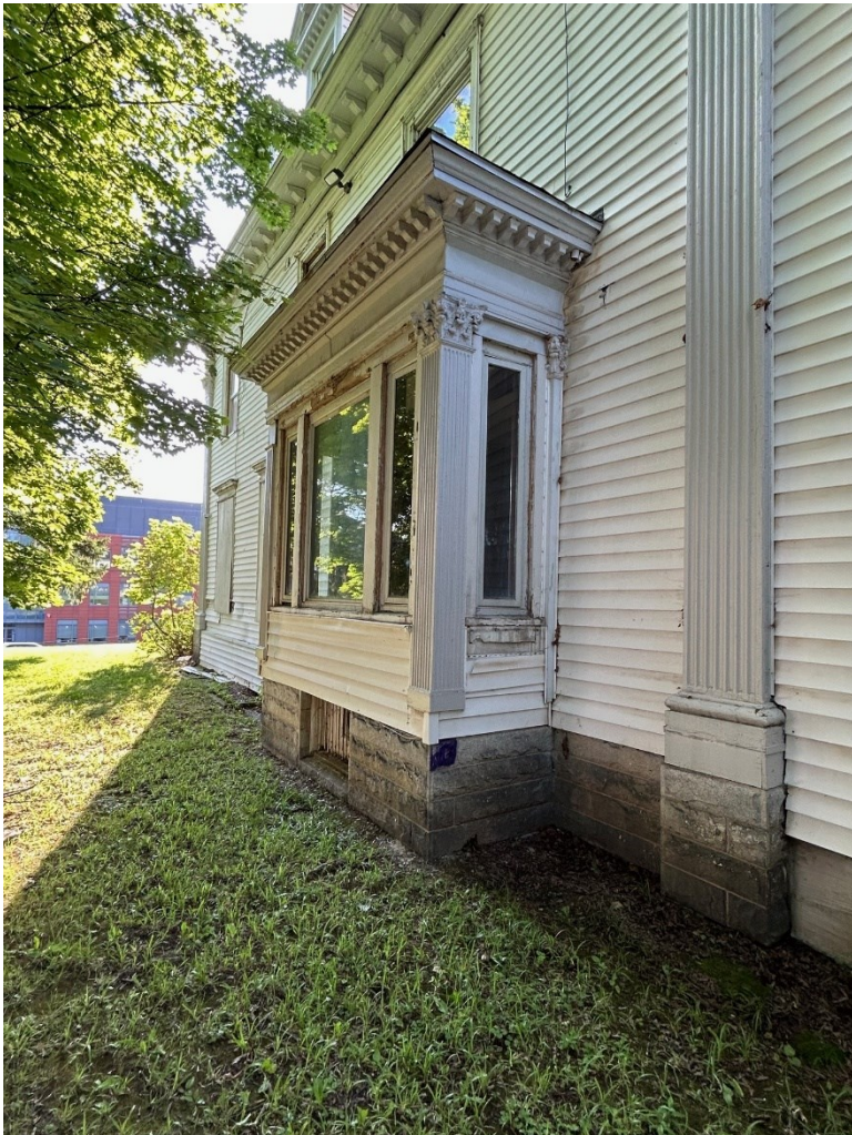
727 Comstock Avenue: South façade, bay window
