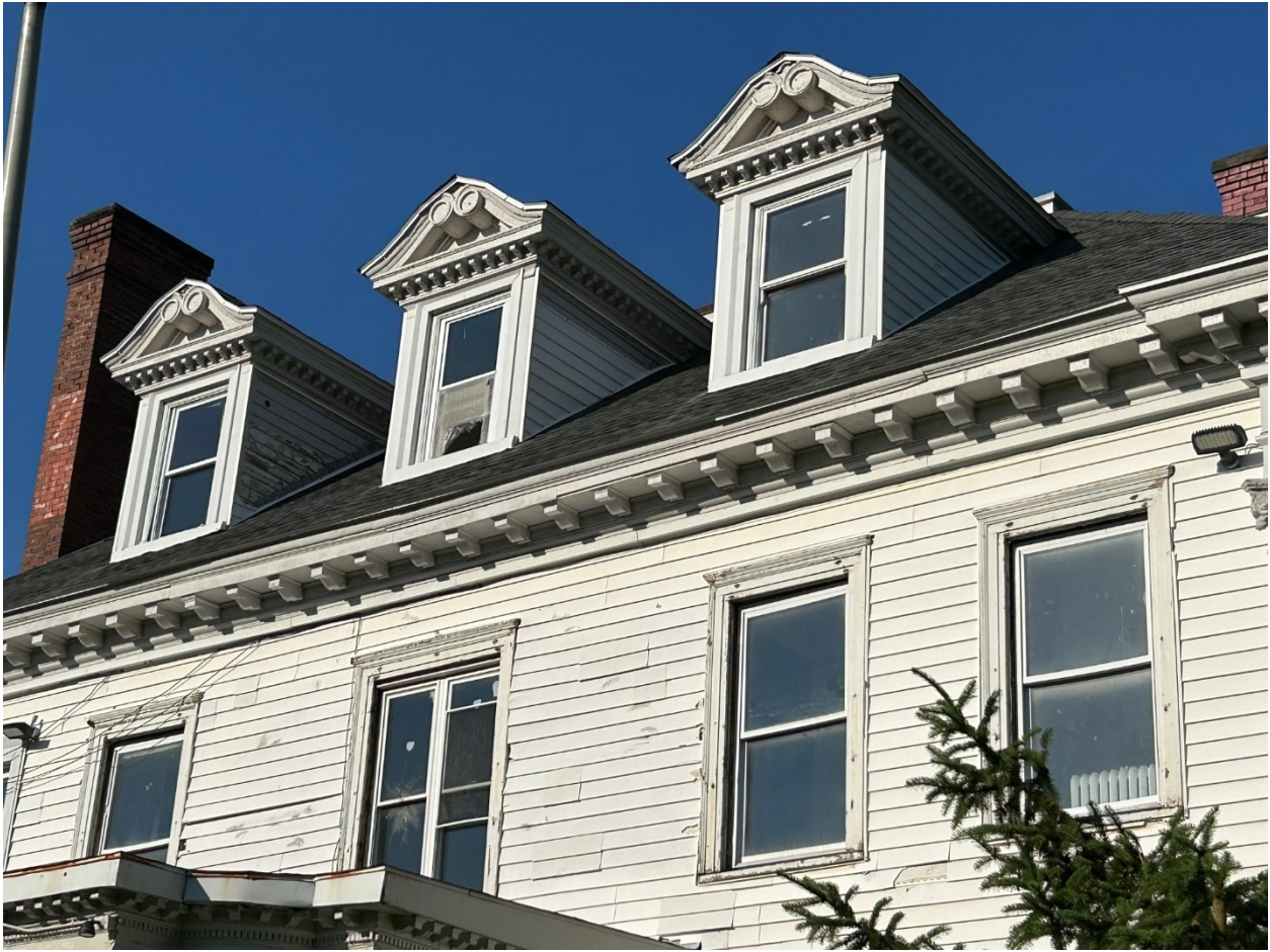
727 Comstock Avenue: West façade, roof dormer detail
