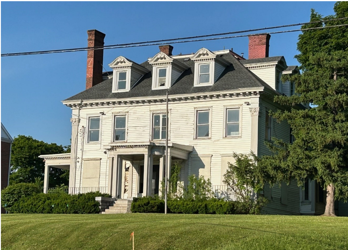
727 Comstock Avenue: West (main) and south facades
