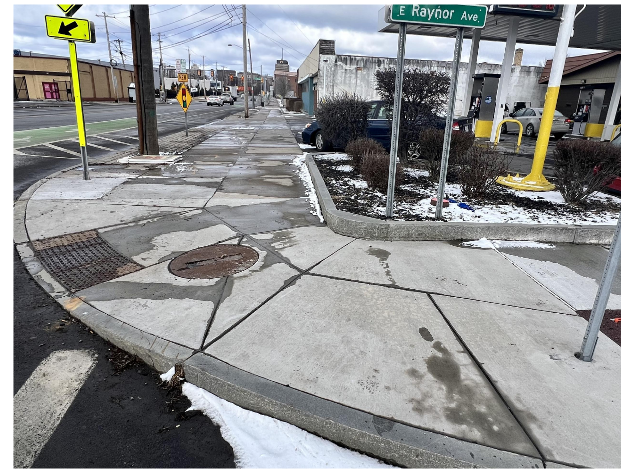
5 EXISTING SITE: VIEW LOOKING NORTH AO.2
