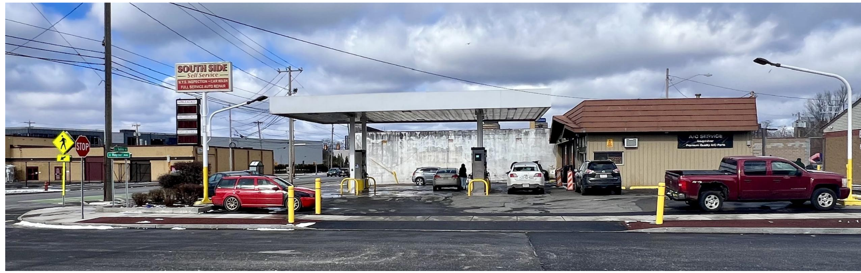
4 EXISTING SITE: VIEW LOOKING NORTH (SOUTH ELEVATION) AO.2
