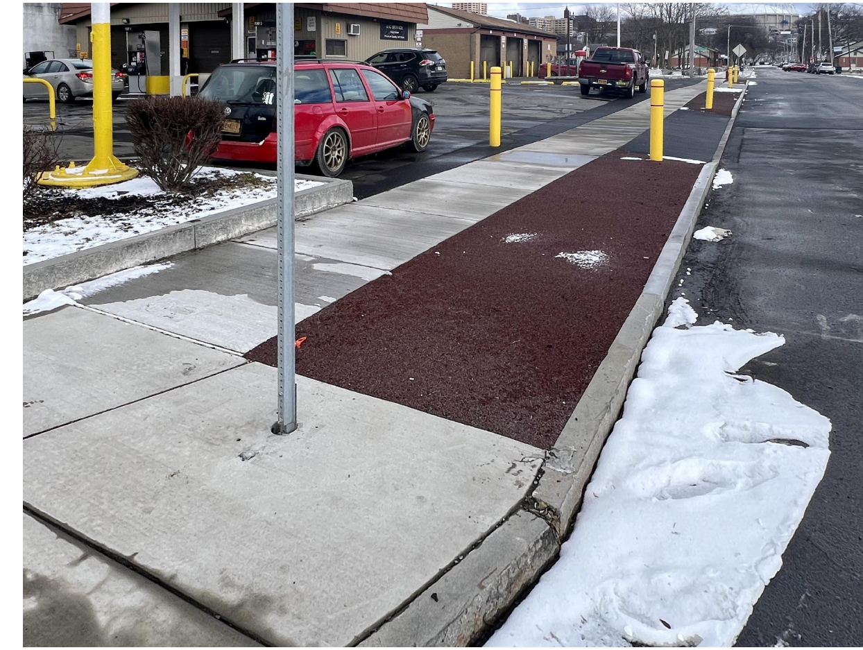
2 EXISTING SITE: VIEW LOOKING EAST AO.2
