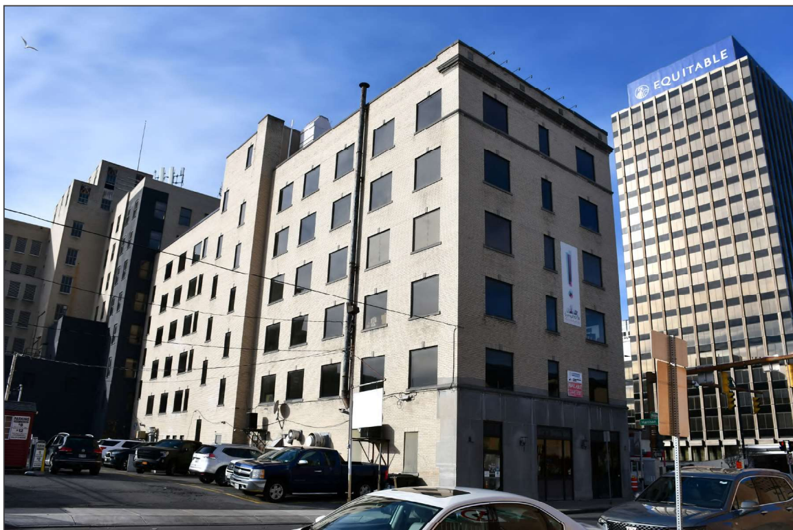
6. South and east elevations, facing northwest
