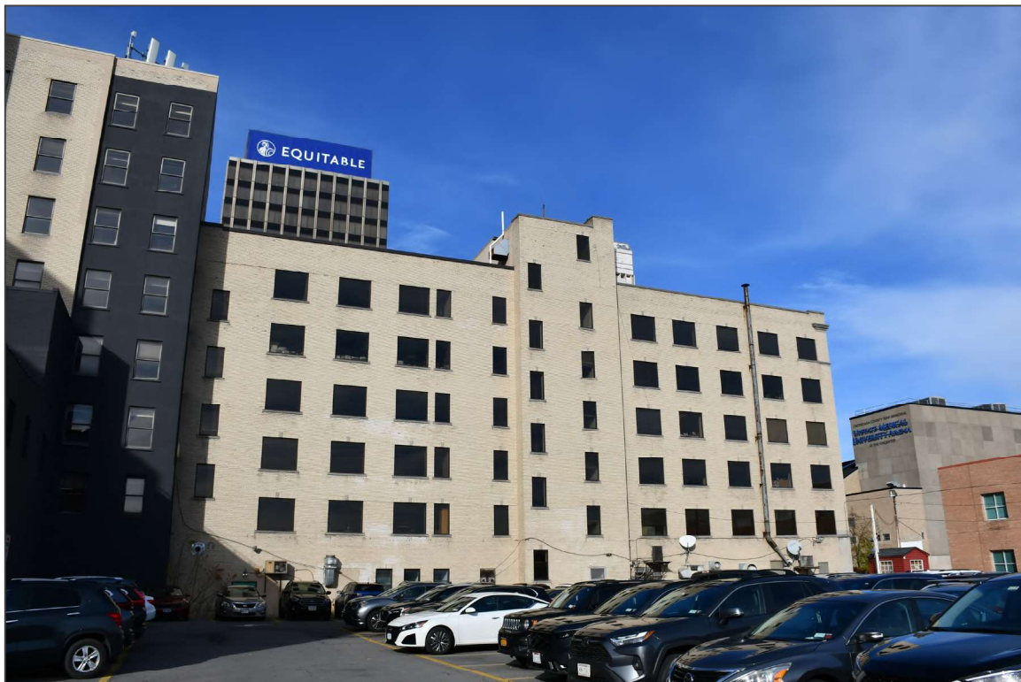
8. South elevation, facing northeast
