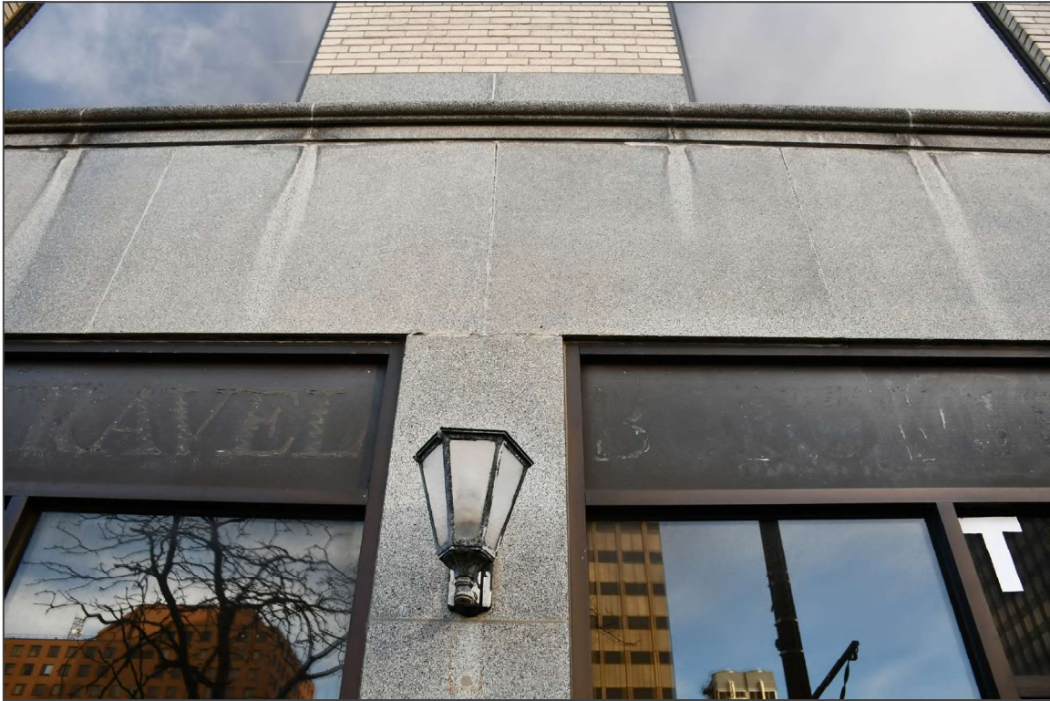
3. North elevation ornamentation detail
