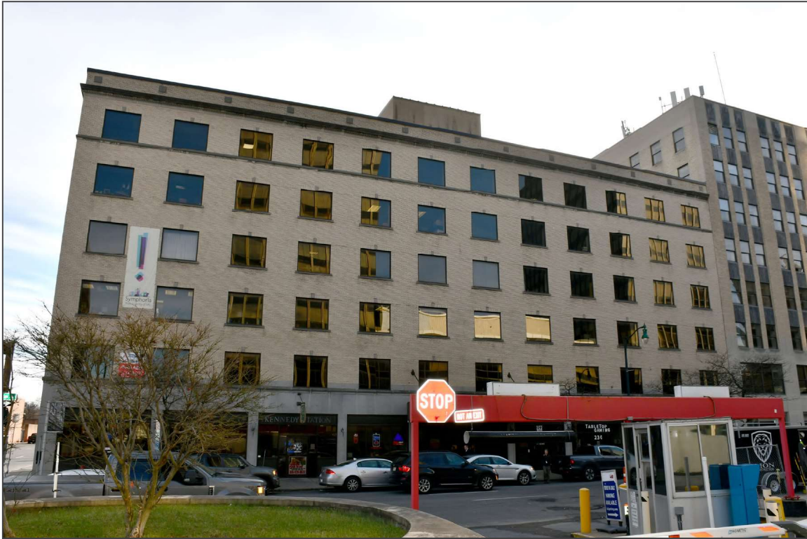
1. North elevation, facing south
