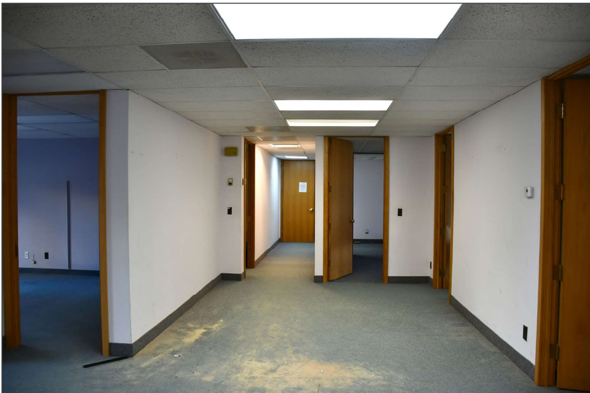
24. Fourth floor, facing east
