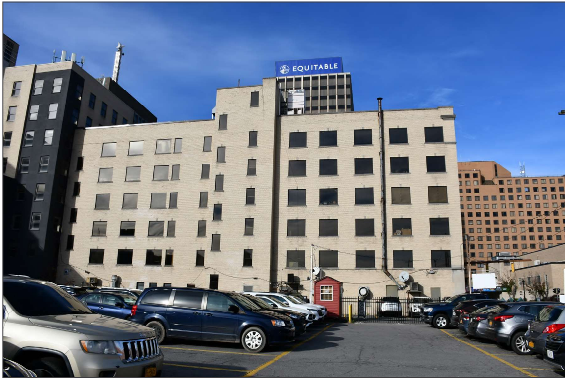
7. South elevation, facing north
