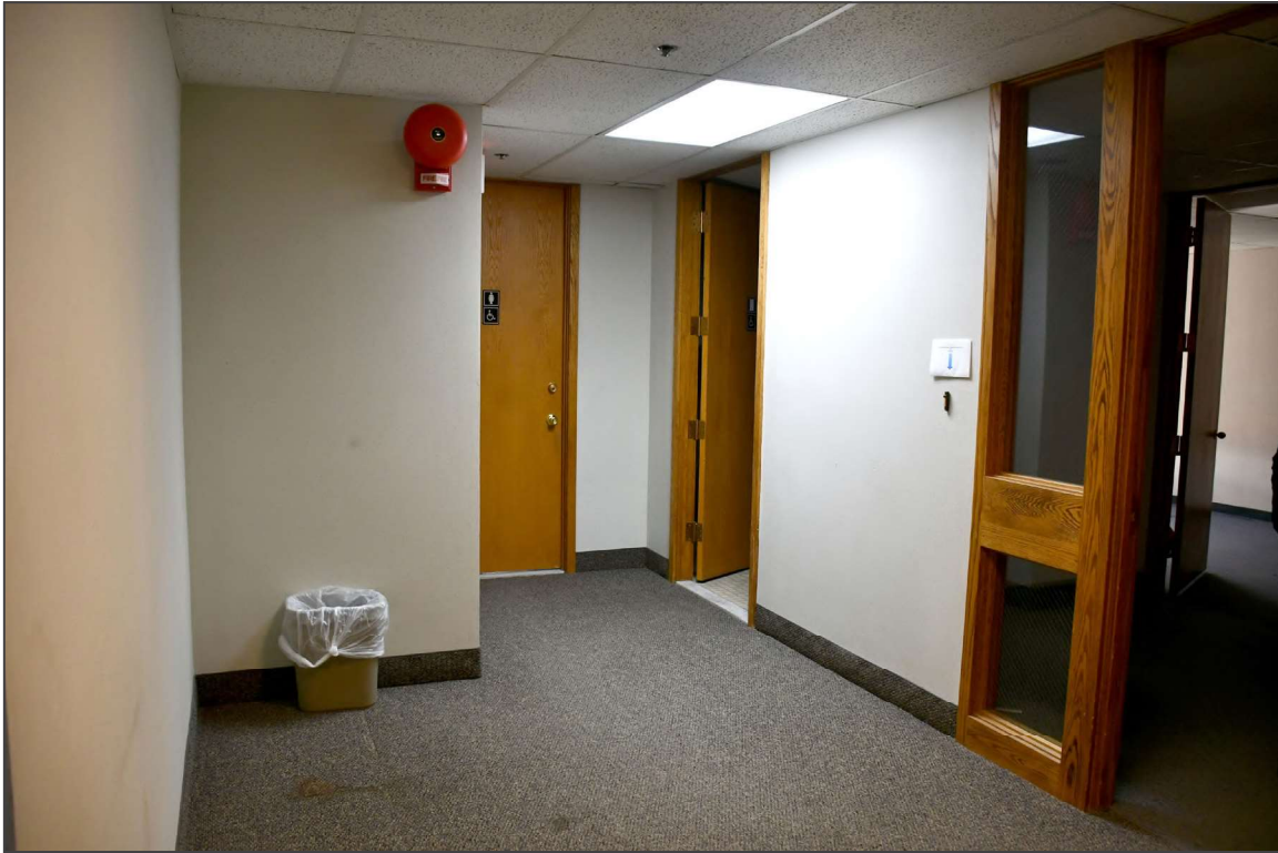
23. Fourth floor, facing southwest
