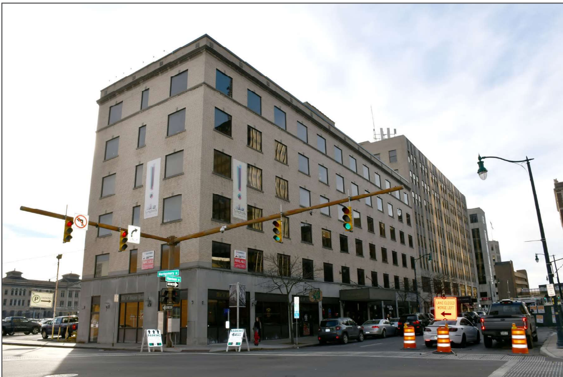
2. North and east elevations, facing southwest
