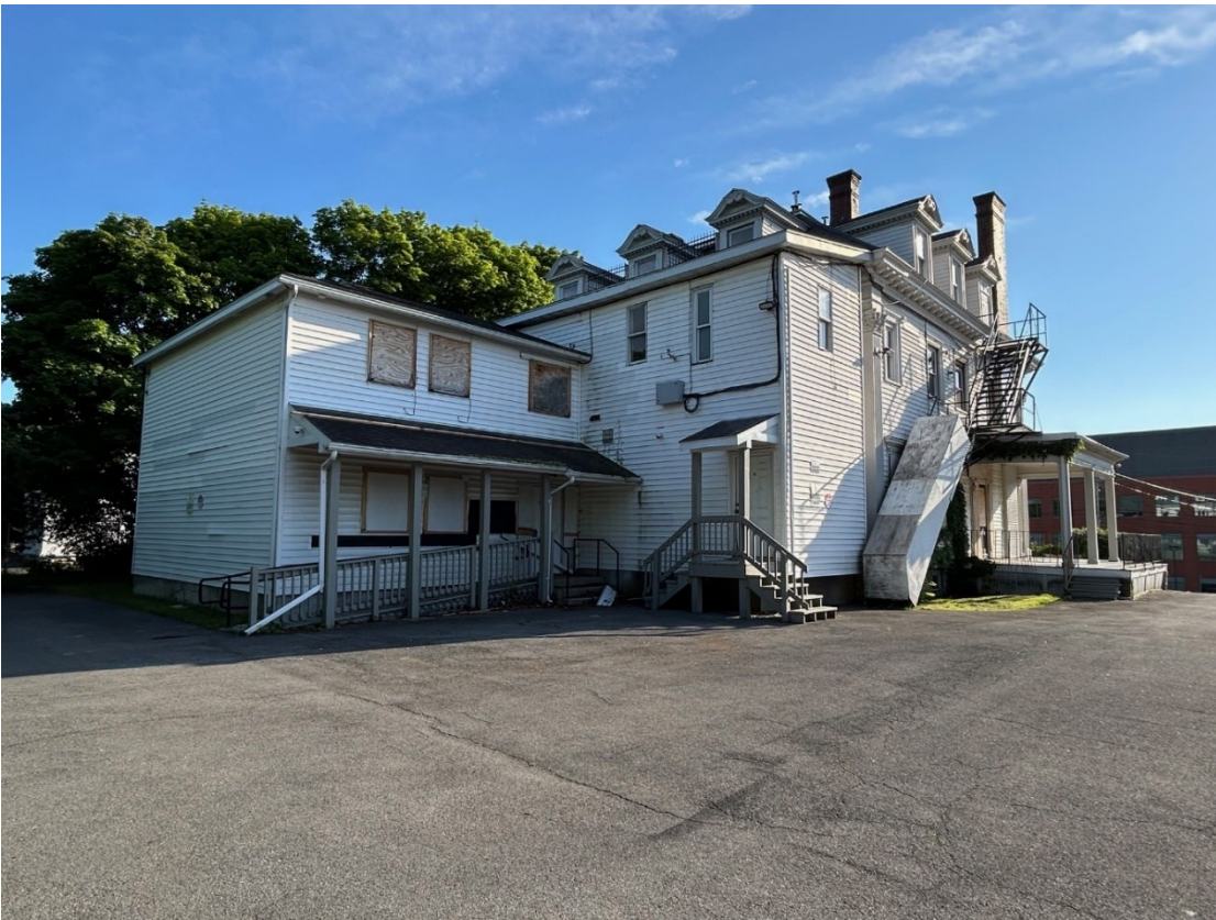
727 Comstock Avenue: North and east facades
