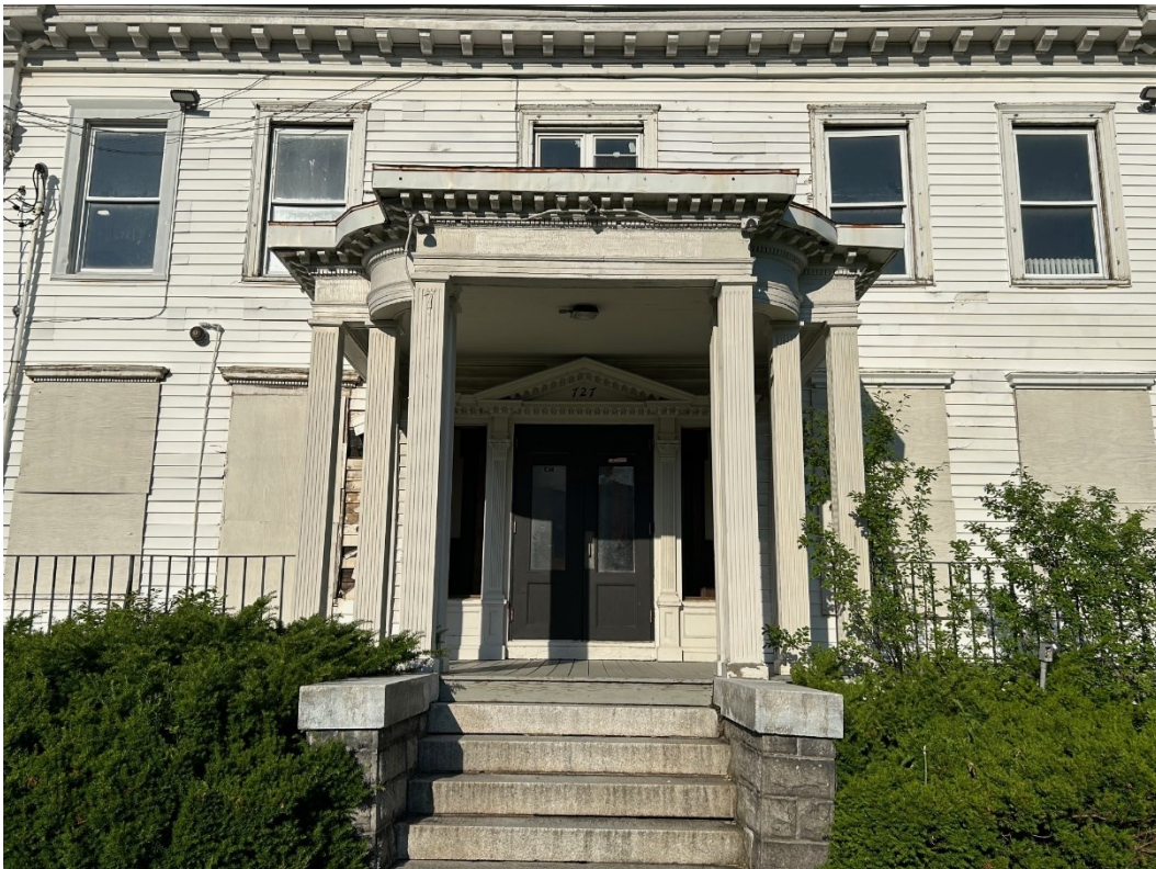
727 Comstock Avenue: West façade, entrance portico
