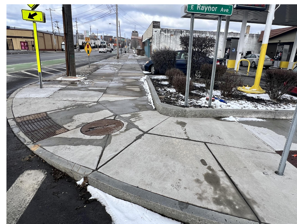
5 EXISTING SITE: VIEW LOOKING NORTH AO.2
