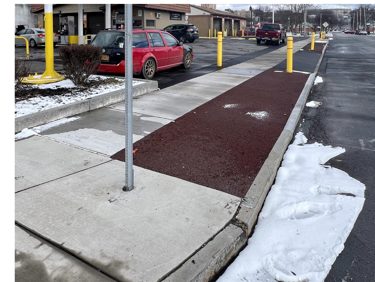
2 EXISTING SITE: VIEW LOOKING EAST AO.2
