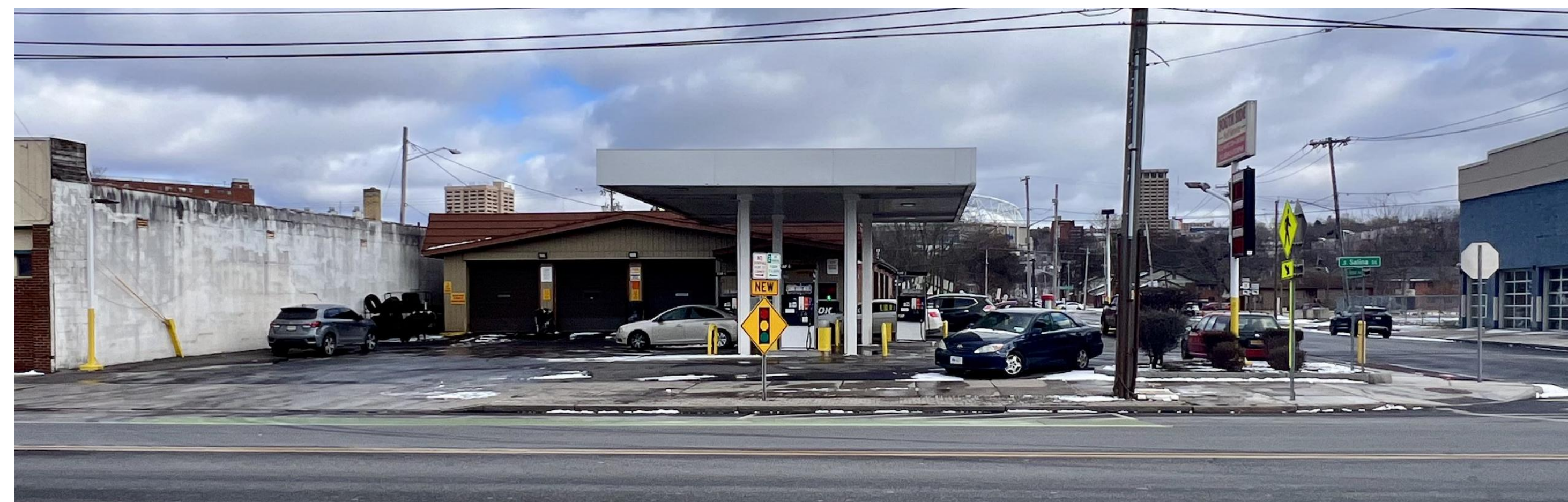
3 EXISTING SITE: VIEW LOOKING EAST (WEST ELEVATION) AO.2
