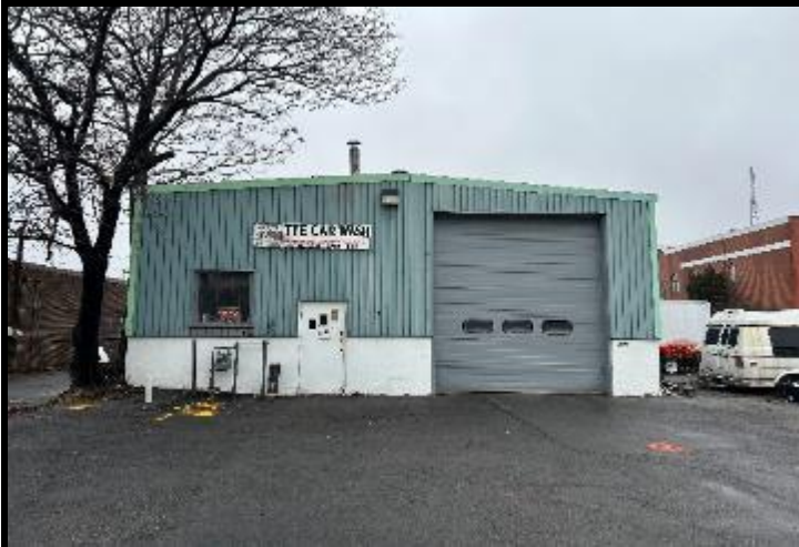
Photograph 7. Autowash exterior looking north.
