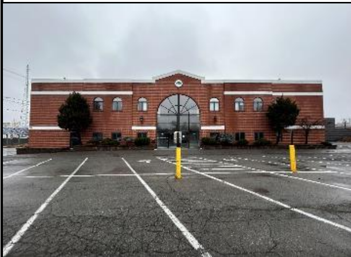
Photograph 9. Vacant office building looking north.
