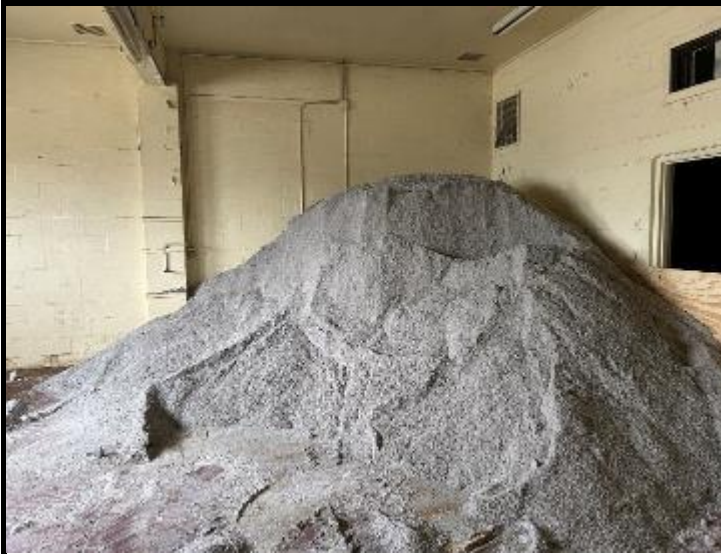
Photograph 13. Pile of salt located inside the abandoned gas station.
