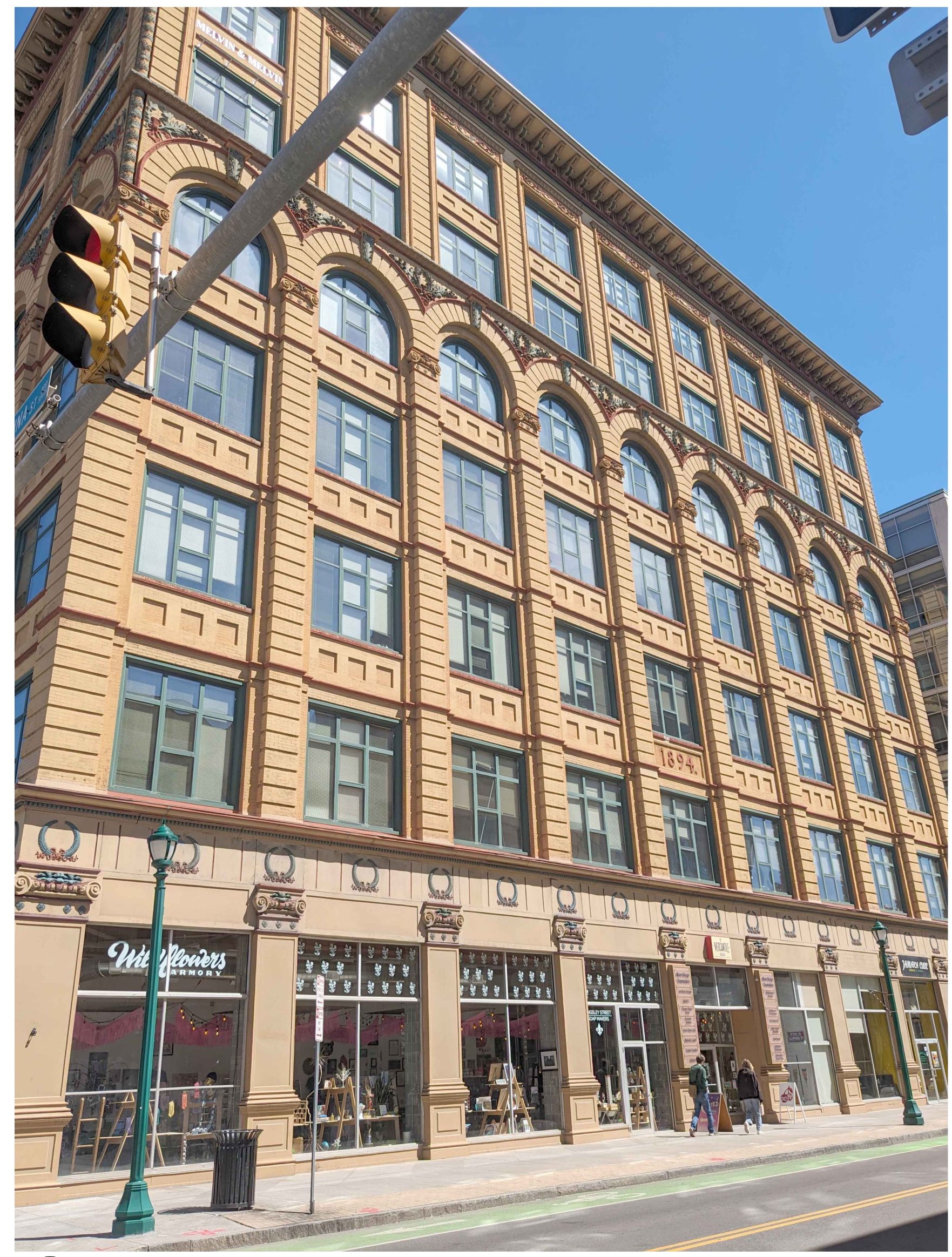
12 EXISTING PHOTO - SOUTH ELEVATION SCALE: NONE
