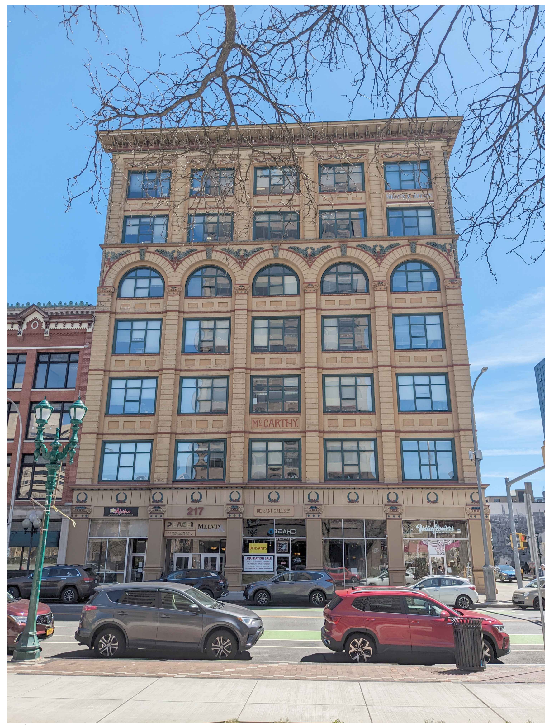
10 EXISTING PHOTO - WEST ELEVATION SCALE: NONE
