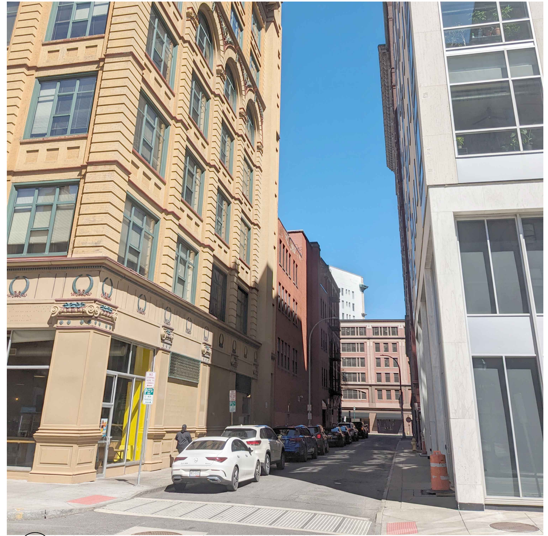
24 EXISTING PHOTO - EAST ELEVATION SCALE: NONE
