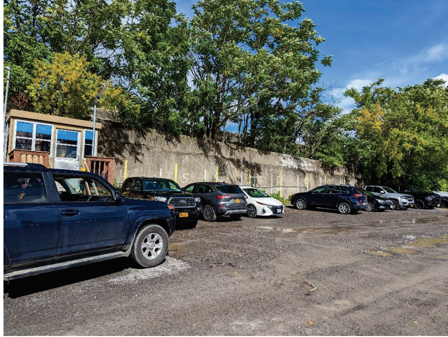
Figure 2 – View of rail line retaining wall at north edge of site
