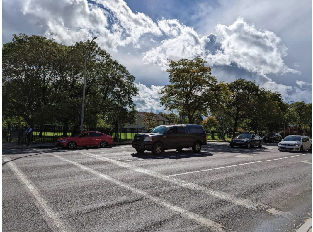
Figure 2 – View of Phase 1 from East Adams Street
