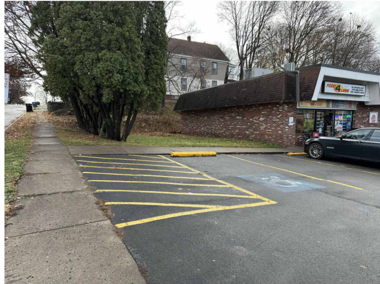
EXISTING ADA PARKING ACCESS.
