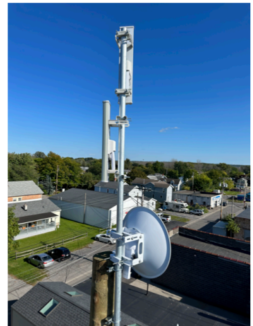
Utility Pole Mounted
