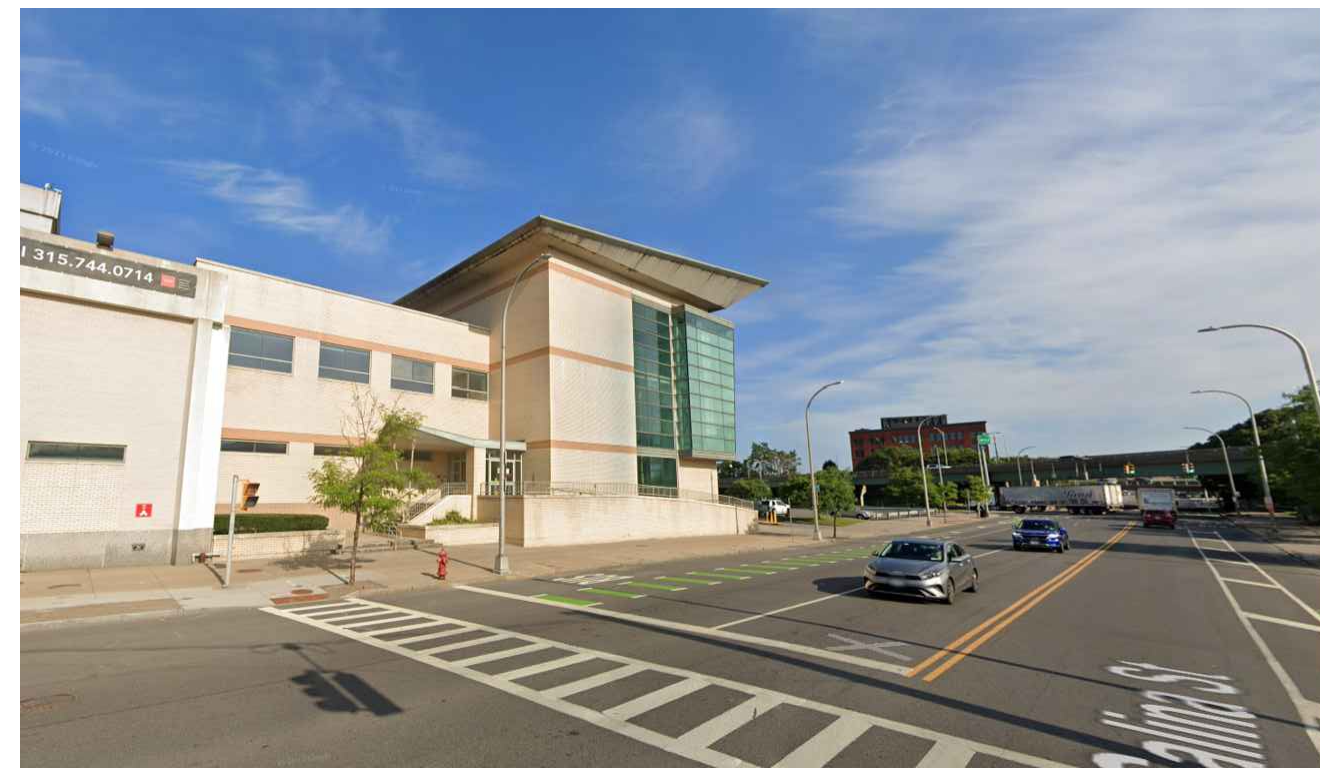
3 RESIDENTIAL ENTRANCE - LOOKING NORTH L-001
