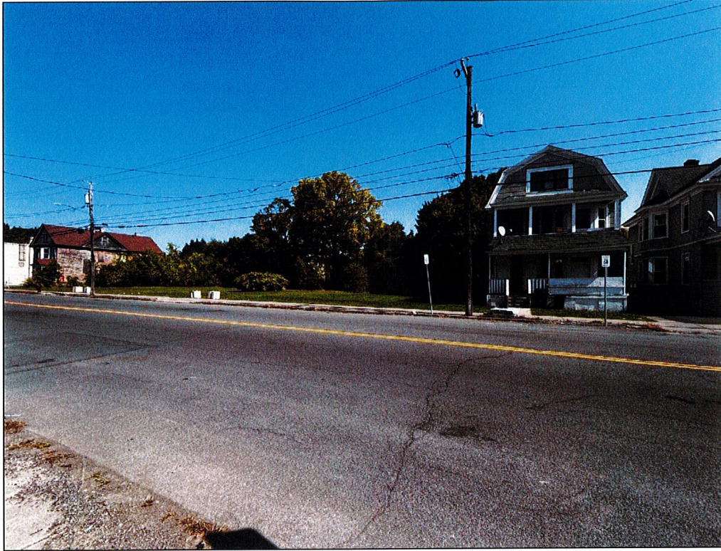
1541-43 South Ave and adjacent vacant lots to the north
