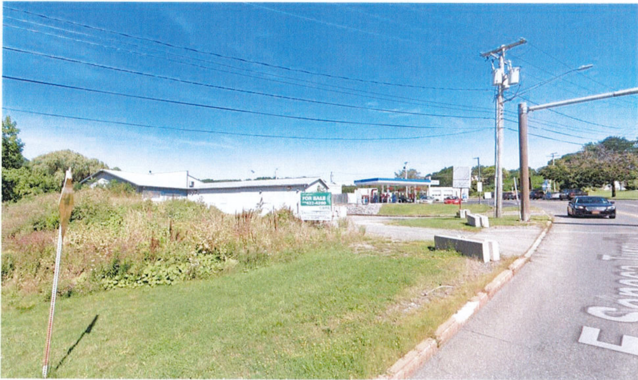
Photograph : From the westerly driveway on E Seneca Turnpike, looking north-east into the site (building to be demolished)
