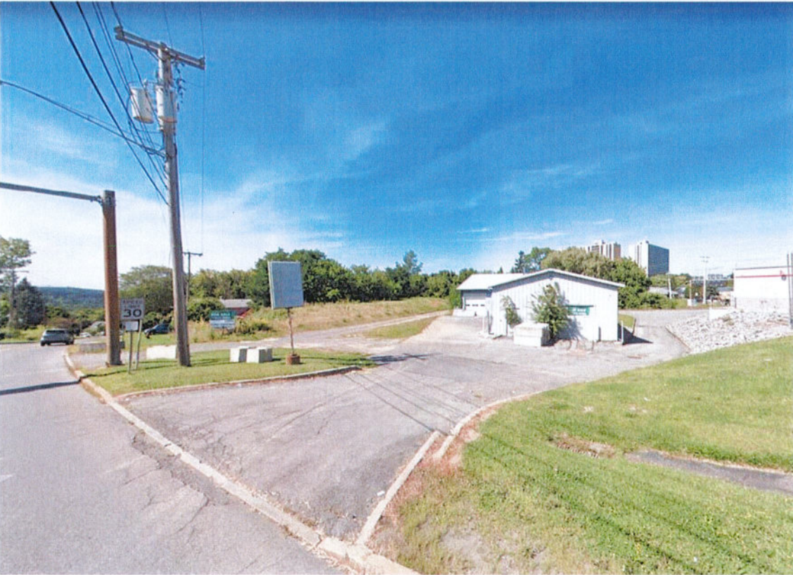
Photograph: From the easterly access drive on E Seneca Turnpike, looking north-west into the subject site (building to be demolished)
