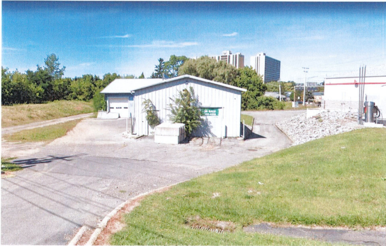
Photograph : From E Seneca Turnpike, looking north (building to be demolished)
