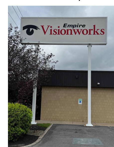
EXISTING CONDITION PHOTO - INFO ONLY
